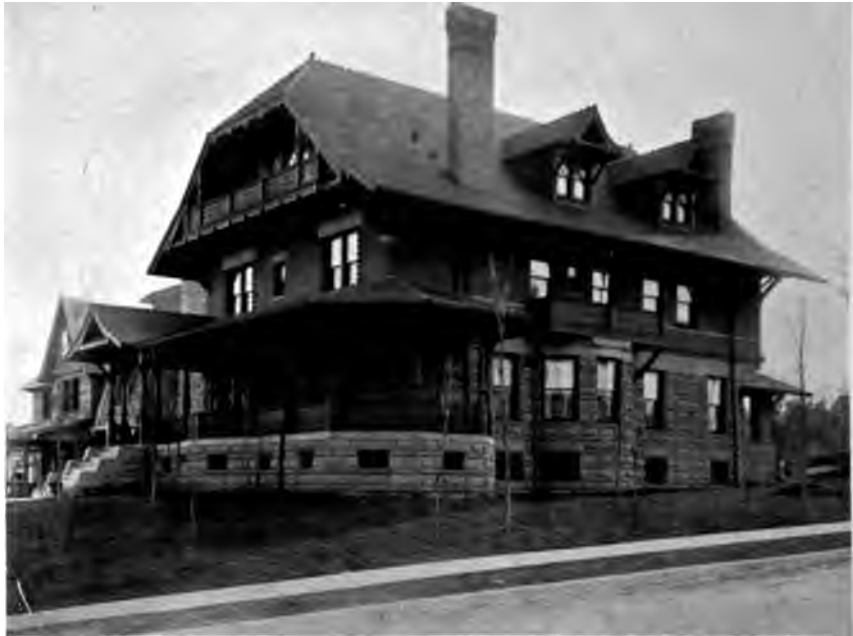
RESIDENCE OF T. H. NOONAN, Avondale, Cincinnati.
